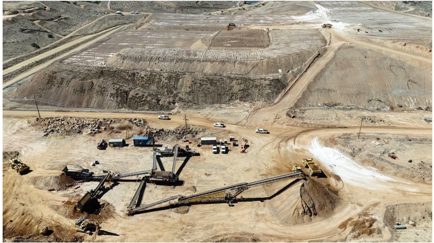
Crushing Spread – March 2026
