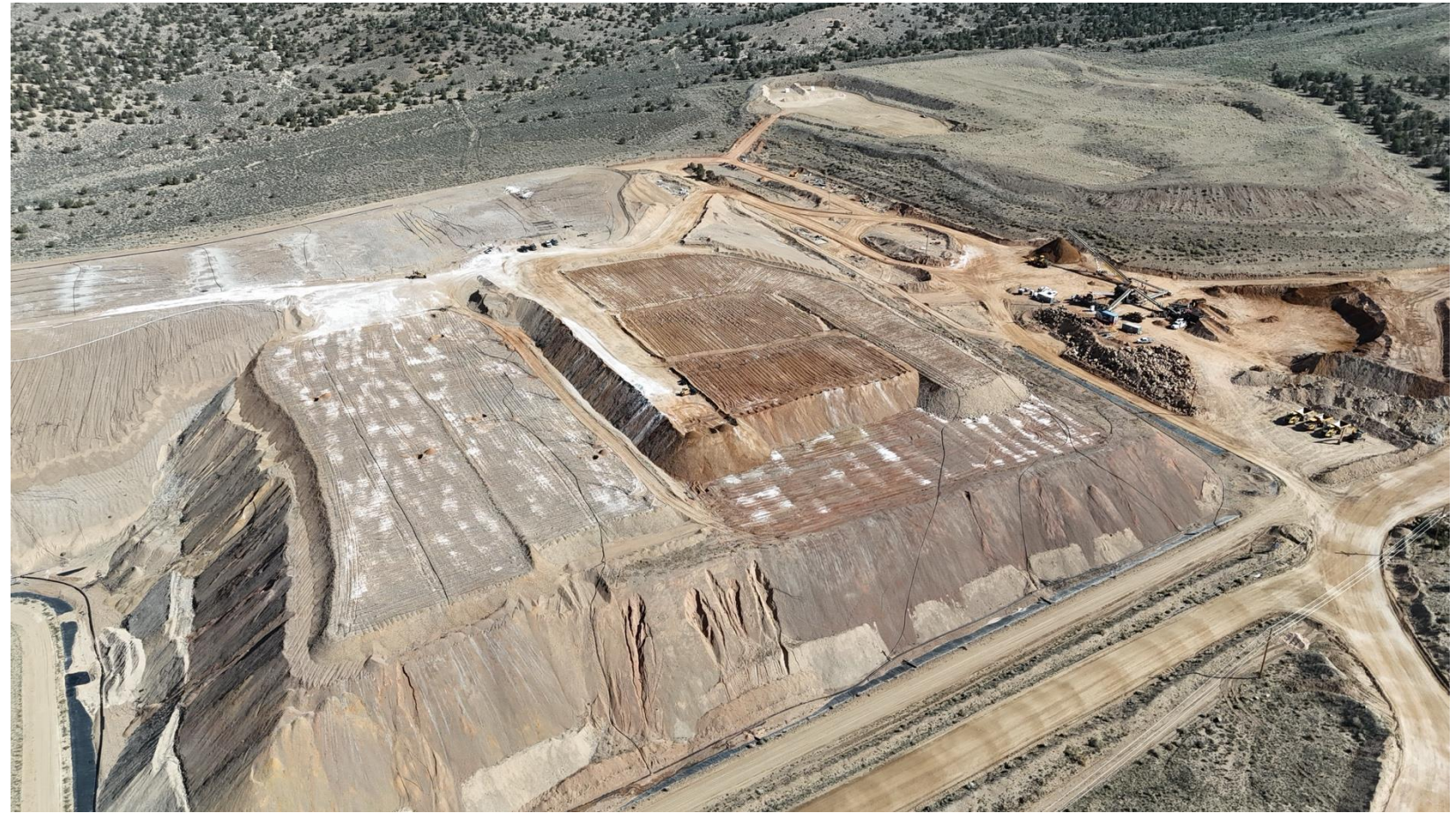
Heap Leach Pad & Crushing Spread – Mid-April 2026
