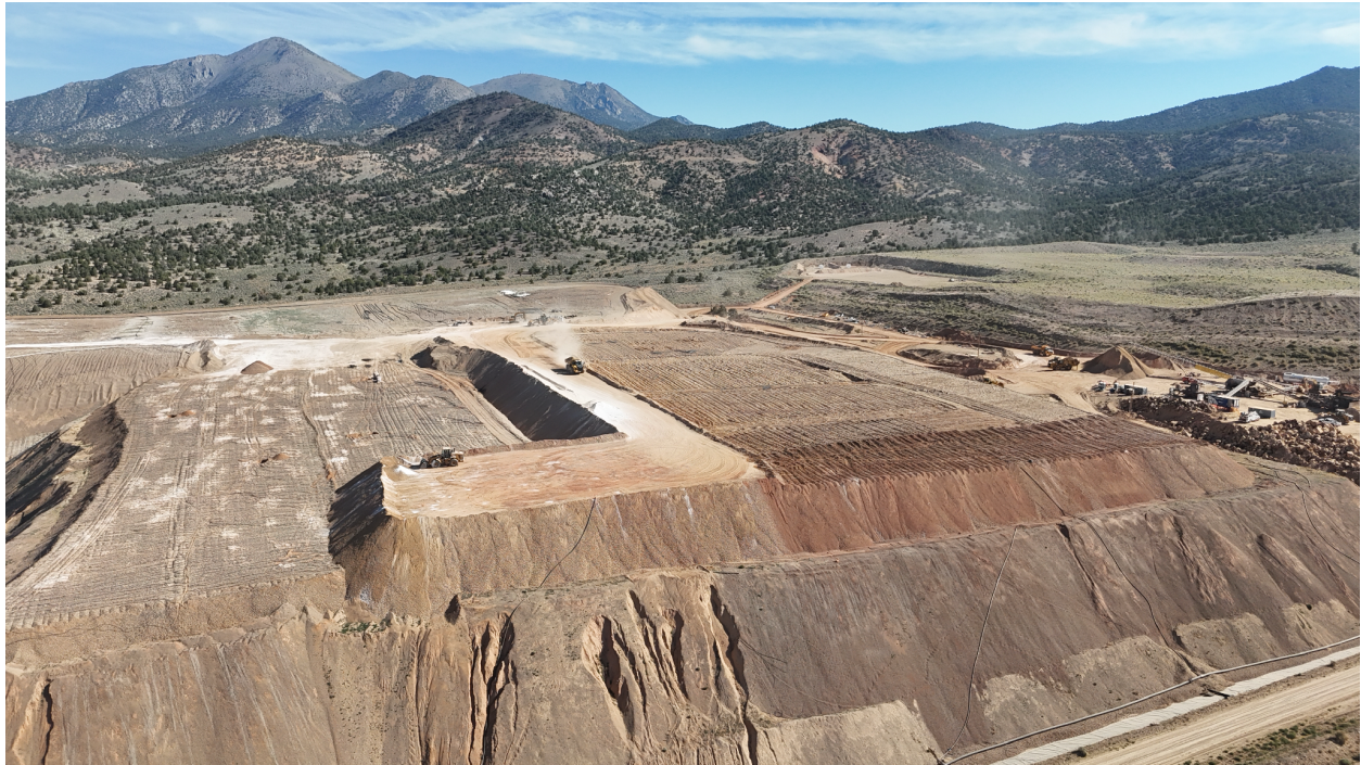
Figure 3 – Heap Leach Pad advancement as at June 16, 2026
