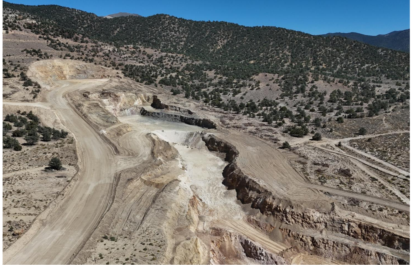
Deep Ore Flats Pit – Newly stripped over past three months
